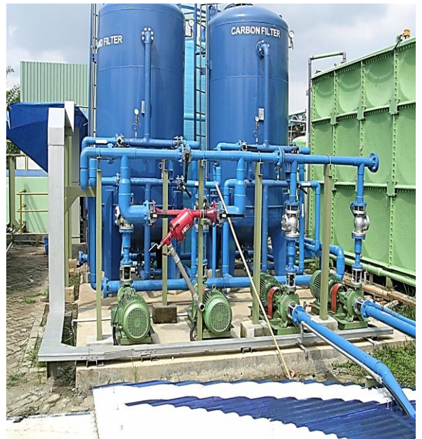
PT. Chemco Harapan Nusantara - Cikarang Carbon & Sand Filter Year construction: 2008 Capacity : 5 m 3 /hour
